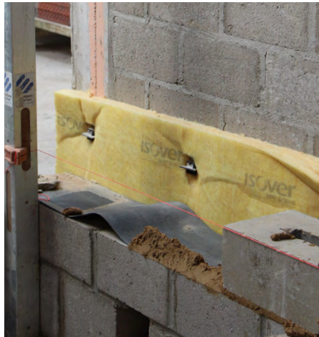
Anti-capillair membraanaanbrengen
