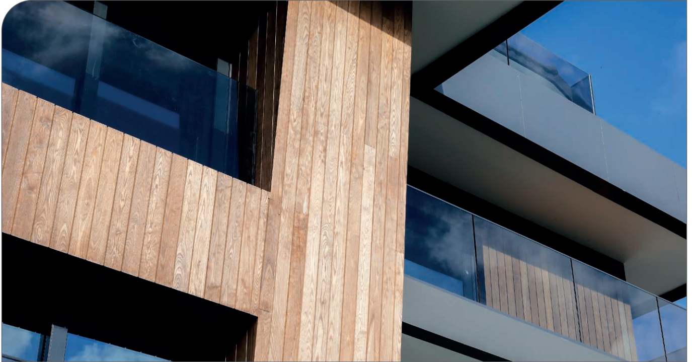
Figure 60. Exterior cladding made of ThermoWood® products. (Turkey).
